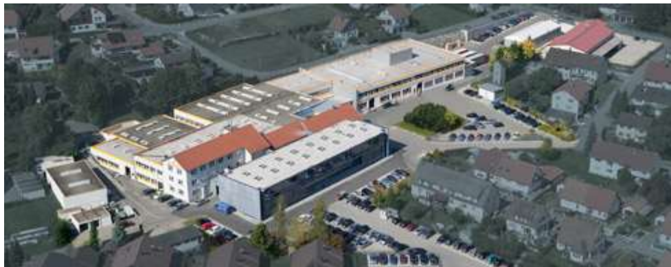
FIGURE 1: AERIAL VIEW OF THE CERTIFIED SITE IN WEHINGEN
